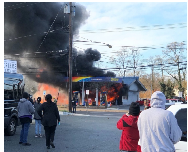
2019 Gasoline Station Fire
