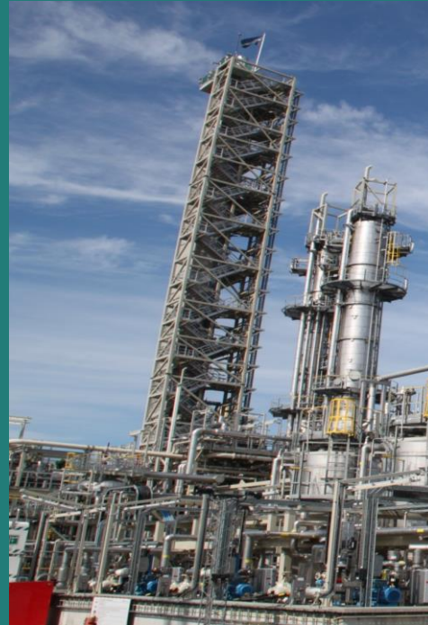
Full-scale validation at Technology Center Mongstad
