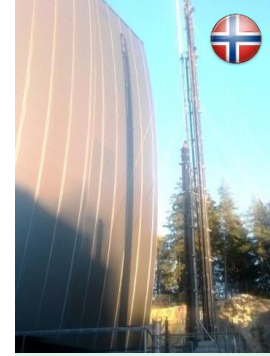
Waste to Energy Klemetsrud WtE
