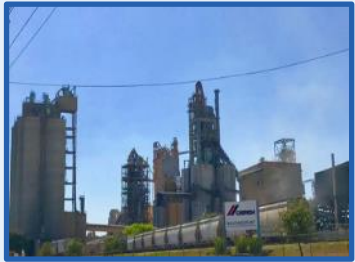
LafargeHolcim Cement Plant Florence, CO
