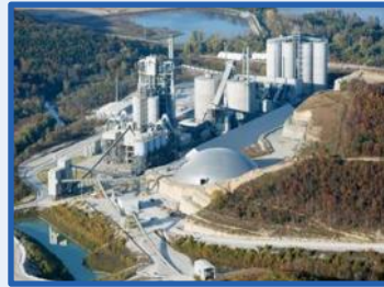
Holcim Ste. Genevieve Cement Plant Bloomsdale, Missouri
