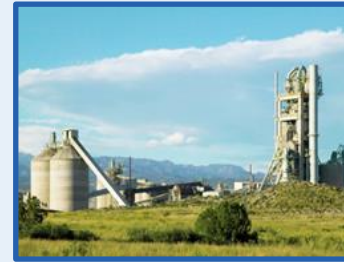
Balcones Cement Plant, New Braunfels, TX
