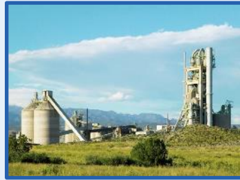
Balcones Cement Plant, New Braunfels, TX
